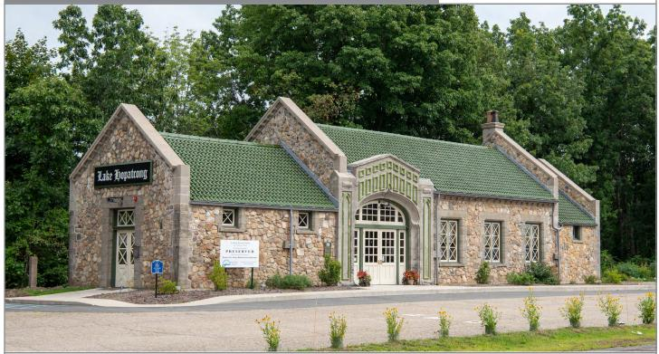
The 1911 Lake Hopatcong Train Station, in Landing New Jersey, was designed to integrate the Morris Canal with rail travel, serving as a link between the two, as well as connecting with adjacent trolley service. The Tudor Revival/Jacobean-style passenger station is of rubble stone and cast stone construction with cast stone detailing and a glazed clay tile roof.
